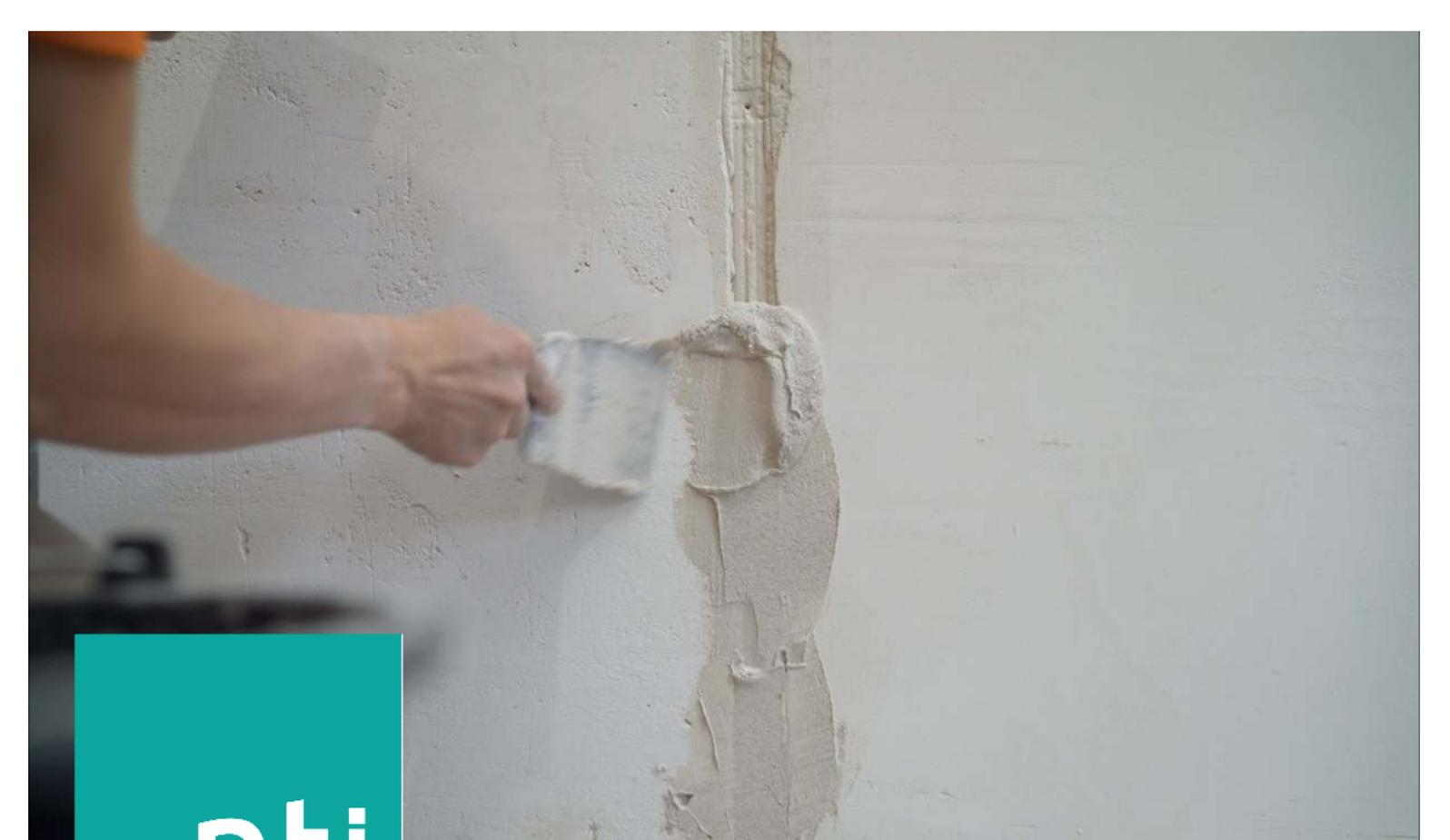
A close-up photograph showing a person's hand using a brush to apply a thick, greyish sealant into a vertical crack in a light-colored wall. The crack is filled with a fibrous material, likely the CSL 465 mentioned in the text. The background is a plain, light-colored wall.
